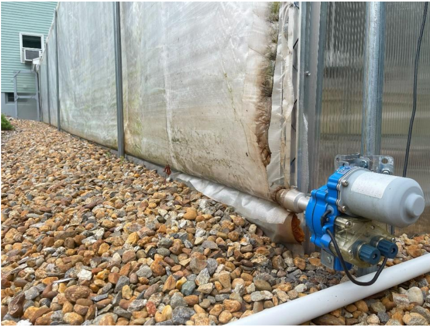
Figure 6. Fully closed side wall with rail seated along base of wall forming its maximum seal.
